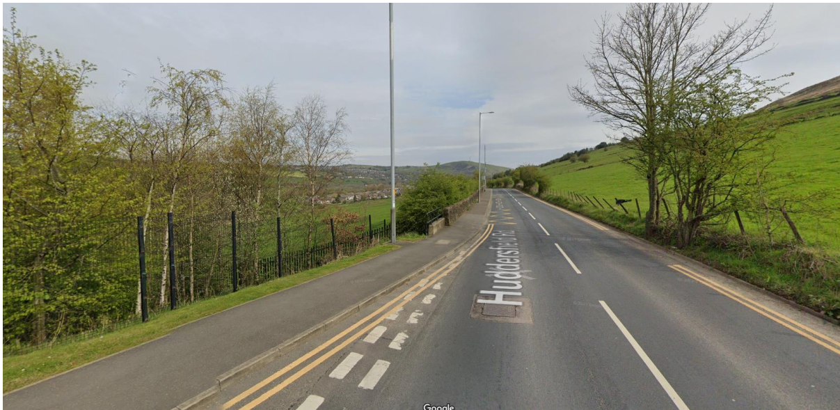
Photo 3: Google Earth image within the vicinity of the proposed site entrance looking North along Huddersfield Road
